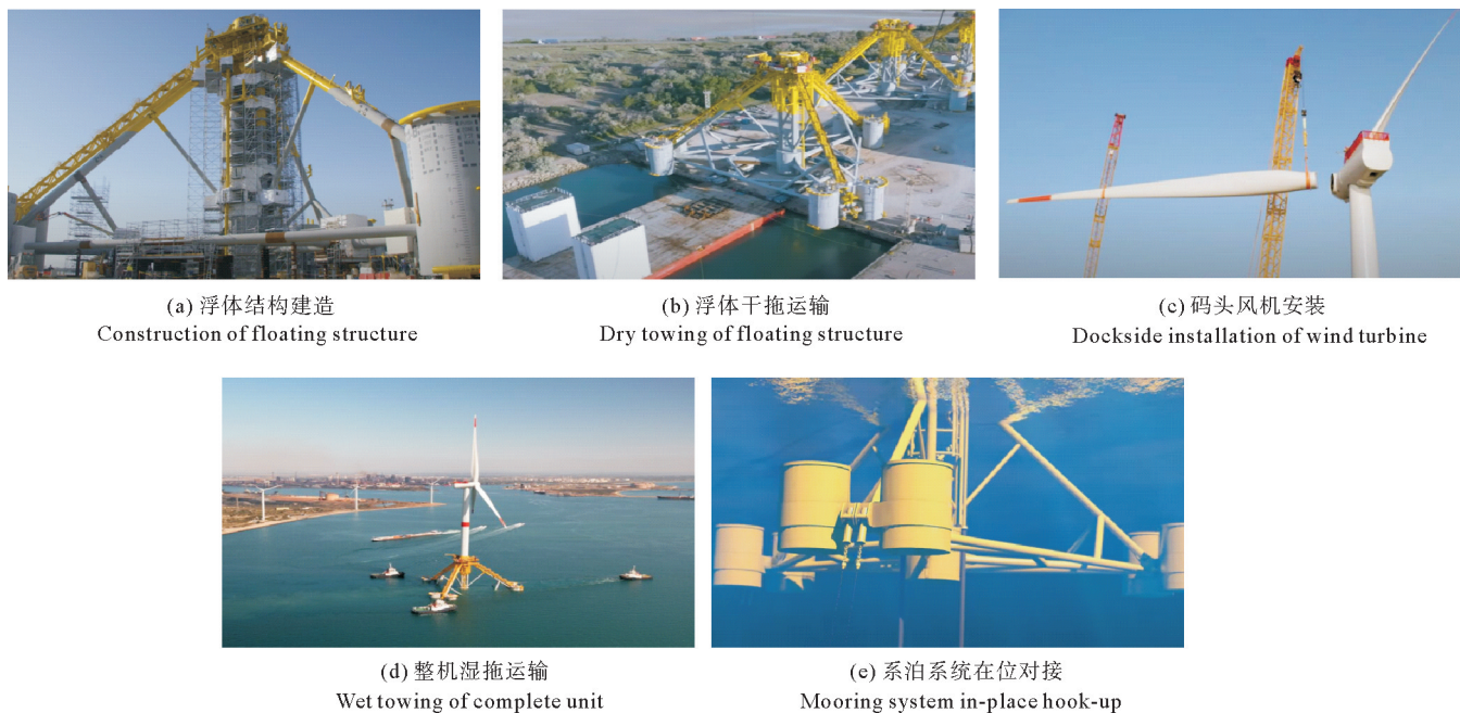
图6 Provence Grand Large 运输和安装作业流程 [29, 37-38] Fig. 6 Construction and installation of Provence Grand Large [29, 37-38]
