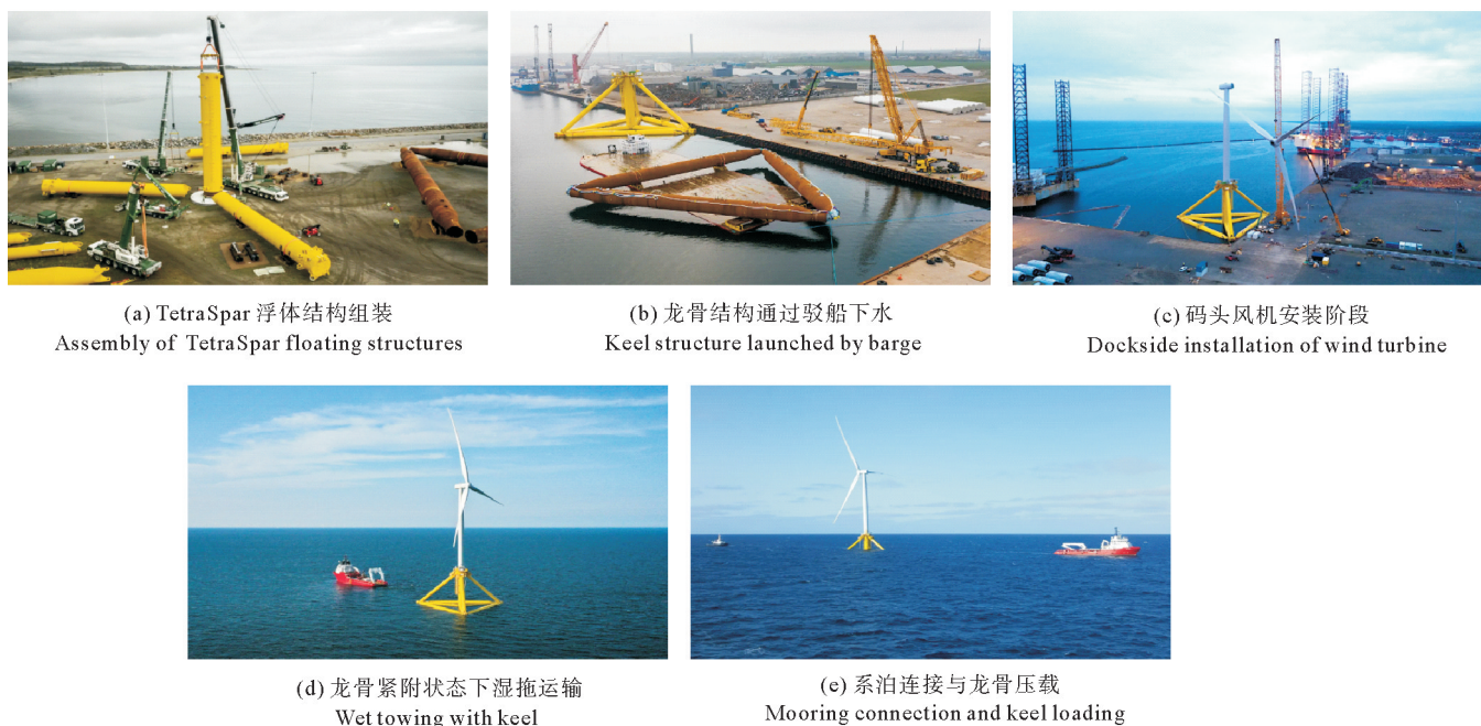
图7 TetraSpar 运输和安装作业流程 [33] Fig. 7 Transportation and installation workflow of TetraSpar [33]
